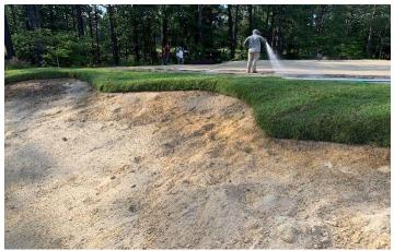
The McDonald and Sons crew is making great progress with the greenside bunkers. They are currently sodding the freshly shaped edges with TifTuf Bermuda grass. This new strand of Bermuda grass was selected due to its superior drought and wear tolerance.
