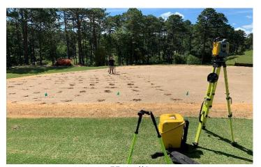
This Robotic Total Station (GPS system) is used to ensure the final grades match the original 3D green scans. The most noticeable change that you will see in the greens complex is that they have returned to their original size. The larger surface will give us more usable pin locations and let's hope more greens in regulation!
