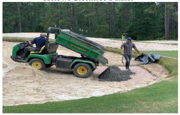
The sump (large drain basin) in each bunker will receive a layer of Capillary Concrete. The porous concrete layer will help deliver more efficient and faster drainage at the low point in the bunker.
