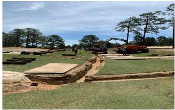
All greenside areas that require shaping and/or drainage must be completed before sprigging the Champion Bermuda grass. The McDonald and Sons crew adds extensive drain lines to the right of the 12th green.
