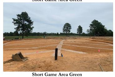
Drainage pipe was added throughout the green and then covered with gravel. The last few steps will consist of adding 10 inches of greens mix, final contours and then sprigging with Champion Bermuda grass.
